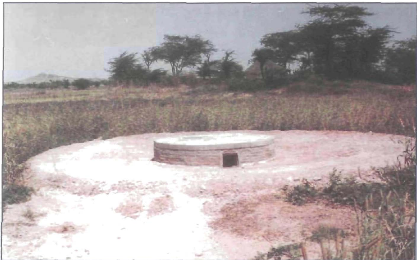
Improved tanka or 21000 liters capacity with catchment at Bambore (Distt. Jodhpur)
