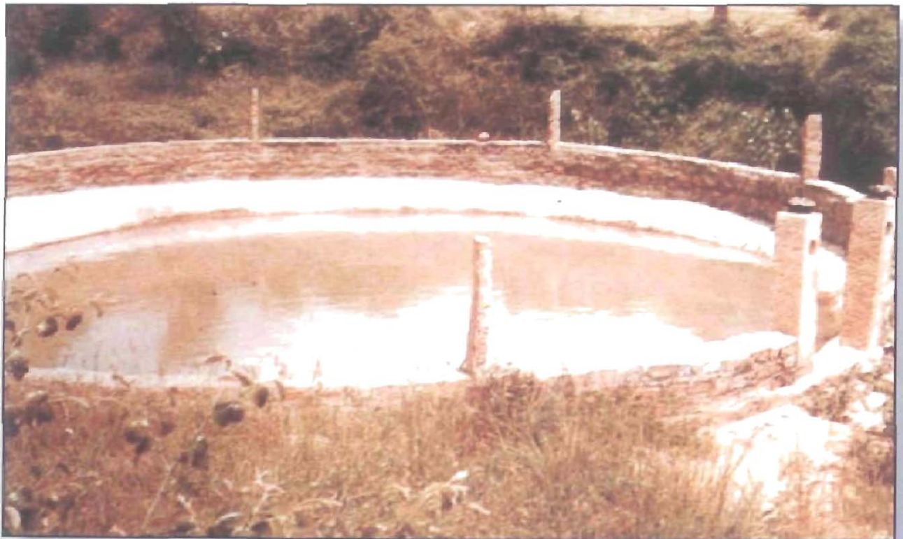
A open tanka of 271 m 3 capacity at farmer's field Jhanwar watershed (Distt. Jodhpur)
