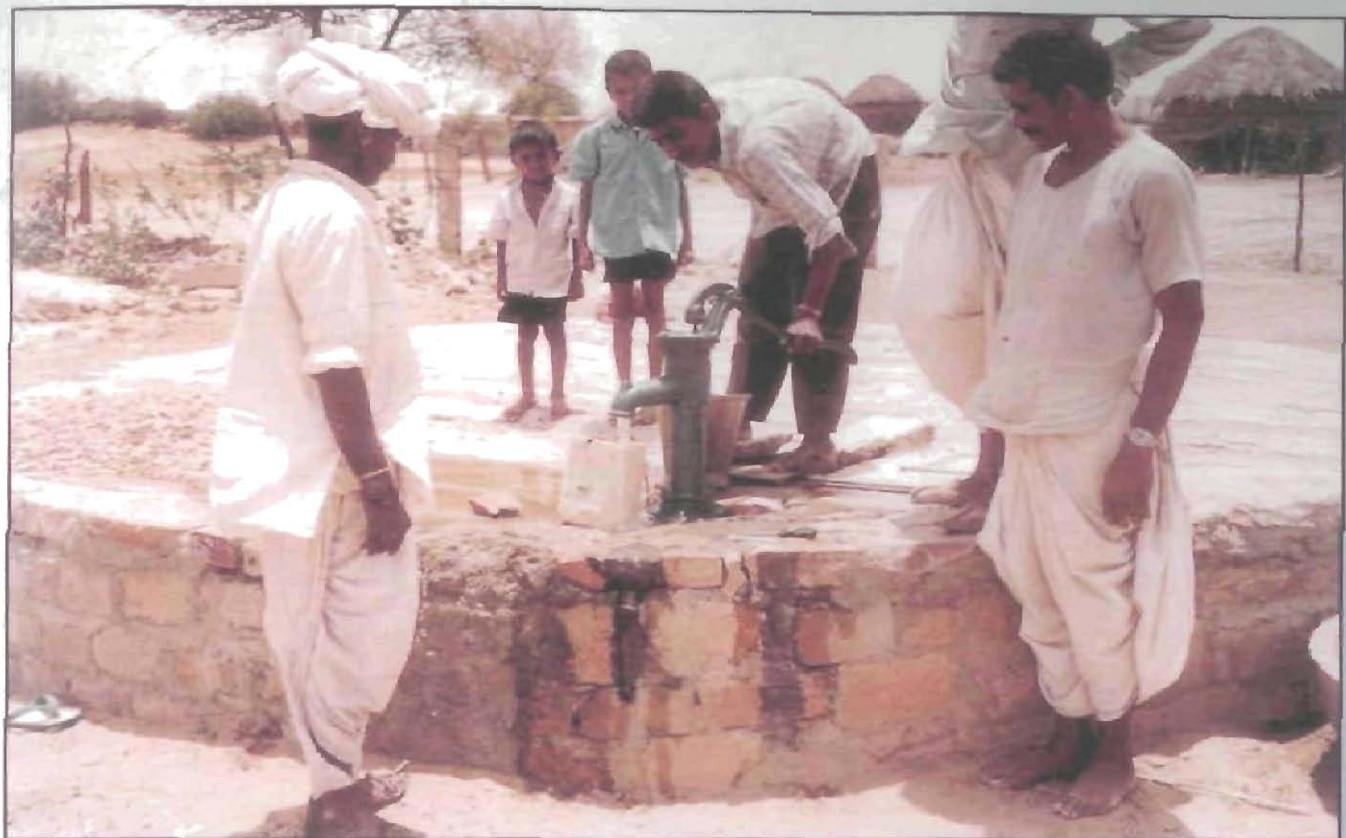
An improved multipurpose tanka (50,000 liters) with handpump for safe water withdrawal at a farmer's field - Kalyanpur (Distt. Barmer)
